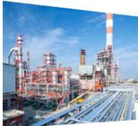
Petroleum and Petrochemical
